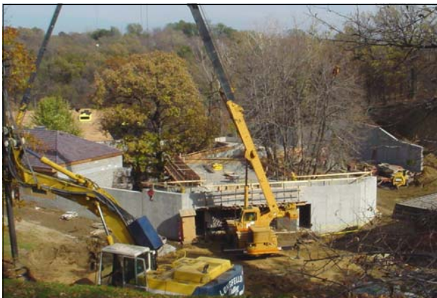
Construction continues on the zoo's Hubbard Gorilla Valley.
